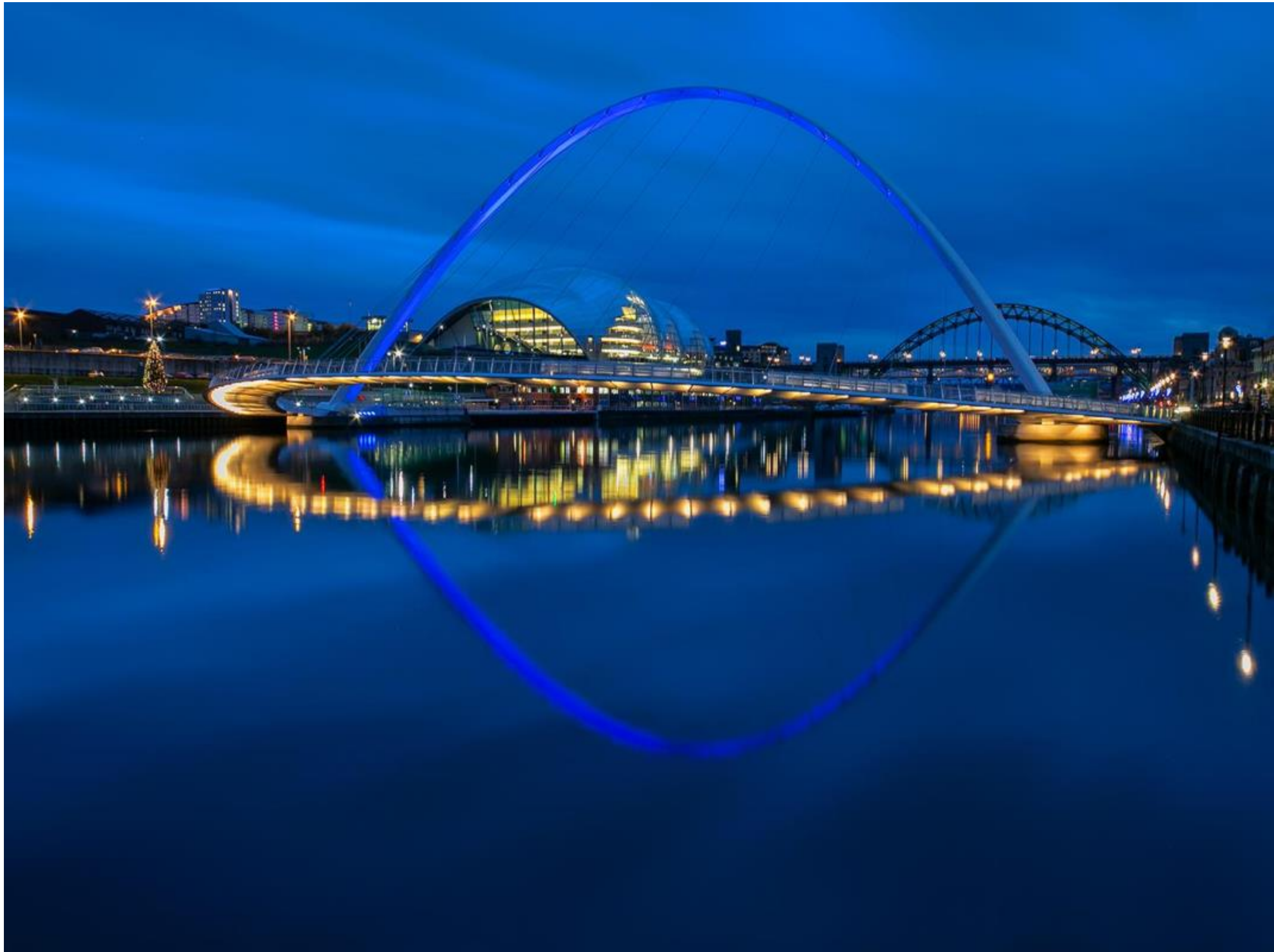
CAPS E-CERTIFICATES - BLUE PHASE ON MILLENIUM BRIDGE by ROBERT MILLIN (ENGLAND)
