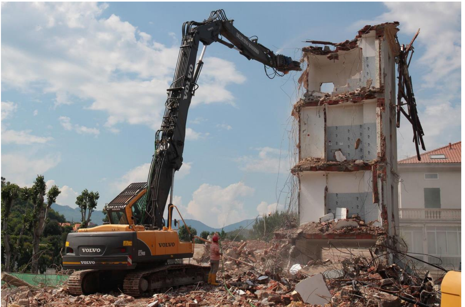
PSA GOLD, TIMELAPSE SILVER - DEMOLIZIONE by EMANUELE ZUFFO (ITALY)
